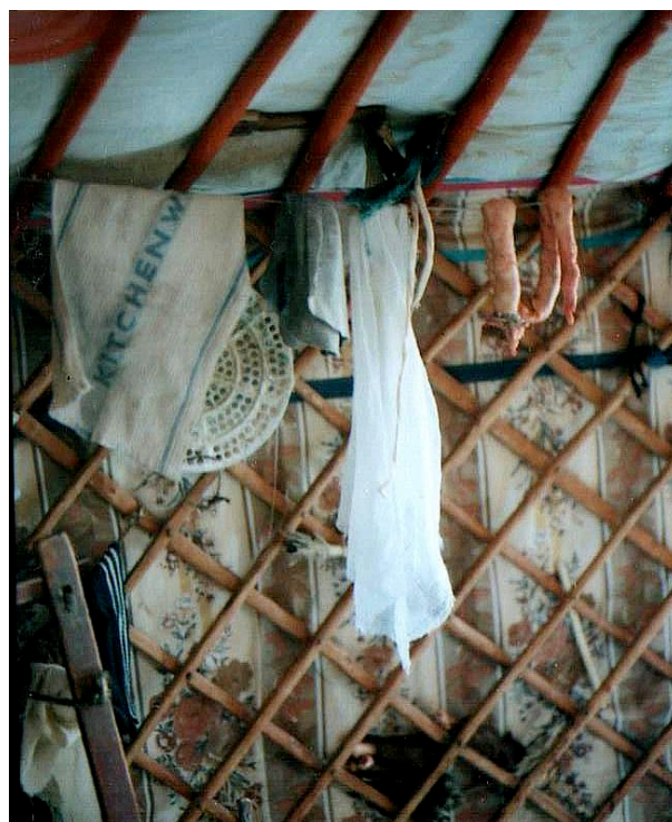
Fig. 20. Trellis wall ( хана ) of a summer ger, showing the lower part of the roof poles ( унь ). Hovd aimag, 2011. (Photograph by author.)
