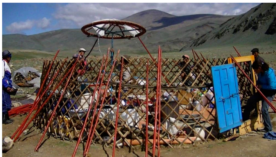
Fig. 22. A ger being taken down at summer’s end: the long outer poles reaching from the tops of the walls to the frame for the roof wheel ( мооно ) have been dismantled, revealing the ‘bristling’ top edge of the circular contractable wall. Khovd aimag, 2011. (Photograph courtesy of Ondřej Srba.)
