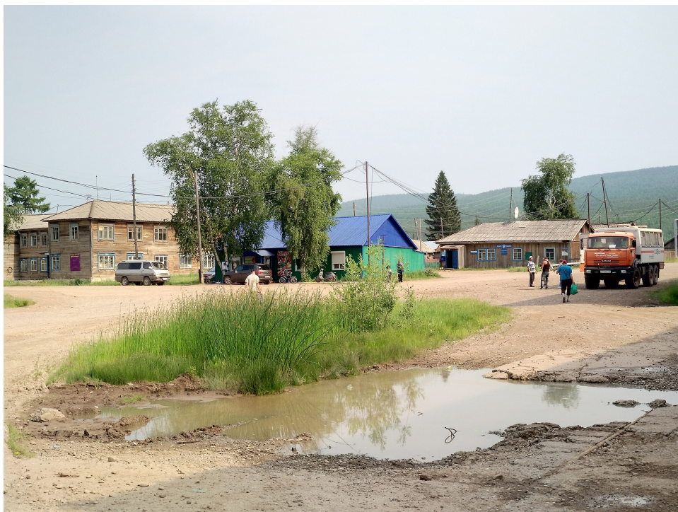
Figure 26.1 The unpaved dirt roads become muddy in spring and fall, central square, Verkhnemarkovo. Photo by G. Saxinger.
